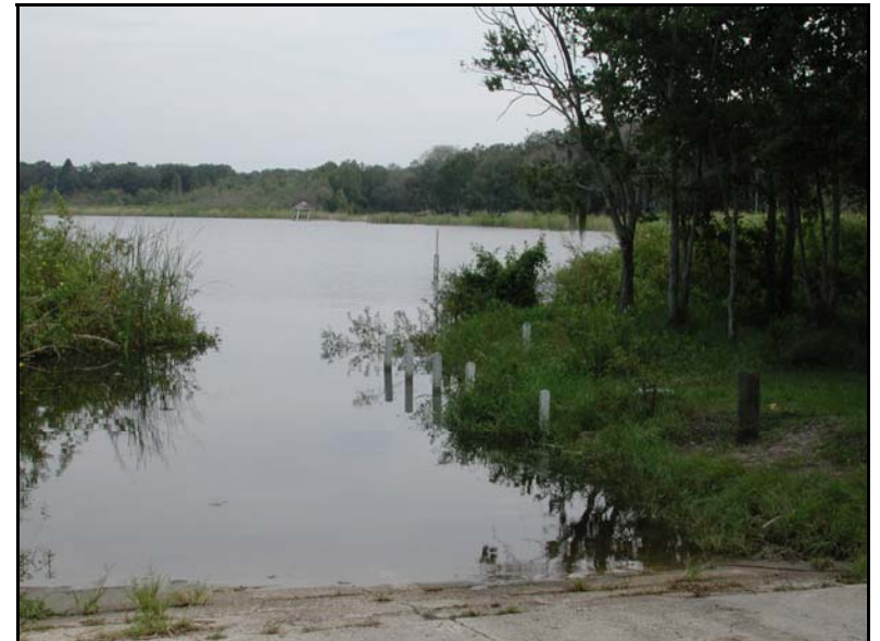
Figure 3 - Vegetation encroaching into boat launch area
